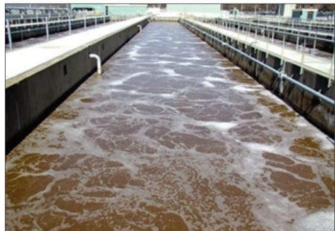
Figure 8: Aeration tank of an activated sludge plant [Available from <http://www.alcosan.org/Education/HowitWorks/HowitWorks2/tabid/95/Default.aspx>]
